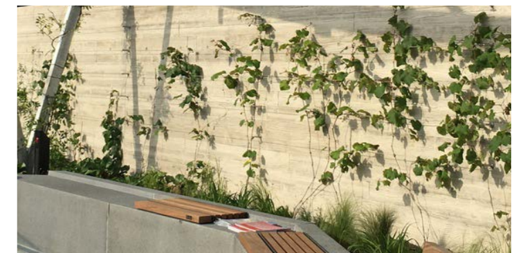
Exposed concrete upper face with strained wire supports for climbing plants.
